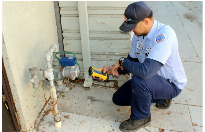
A Long Beach Energy Resources field technician uses a handheld device to communicate with a gas SmartPoint.
